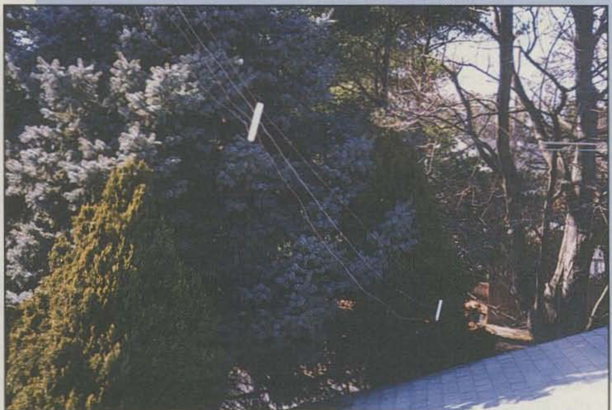
Photo C- This detail of the antenna leg heading toward the front yard shows the different length elements plus the author's redone spreaders.
